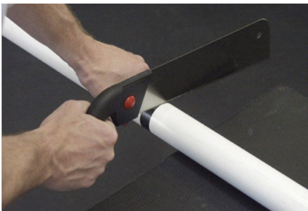
Above: Fine tooth hack saw makes easy work of cutting the pipe.
